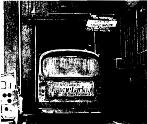
It only takes about a minute to wash the day's grime from Transit coaches with the new automatic racks installed at Atlantic. Each bus is now washed daily.
