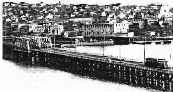
A northbound Puget Sound Traction car crosses the temporary Stoneway Bridge which alternated with the Fremont span until the permanent one was finished in 1917.
