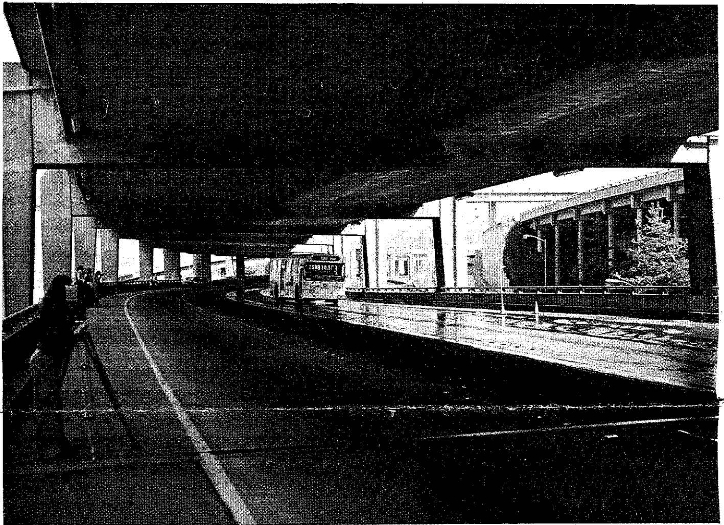
TV crews were on the scene during last month's tests on the I-5 express lanes.
