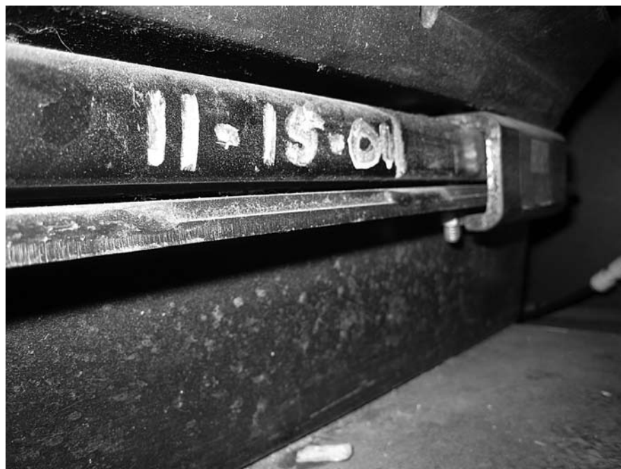
Instead of overhauling this seat with petrified padding, the frame rails were rotated to hide the 2004 overhaul date in the small space between the seat and coach interior wall.
