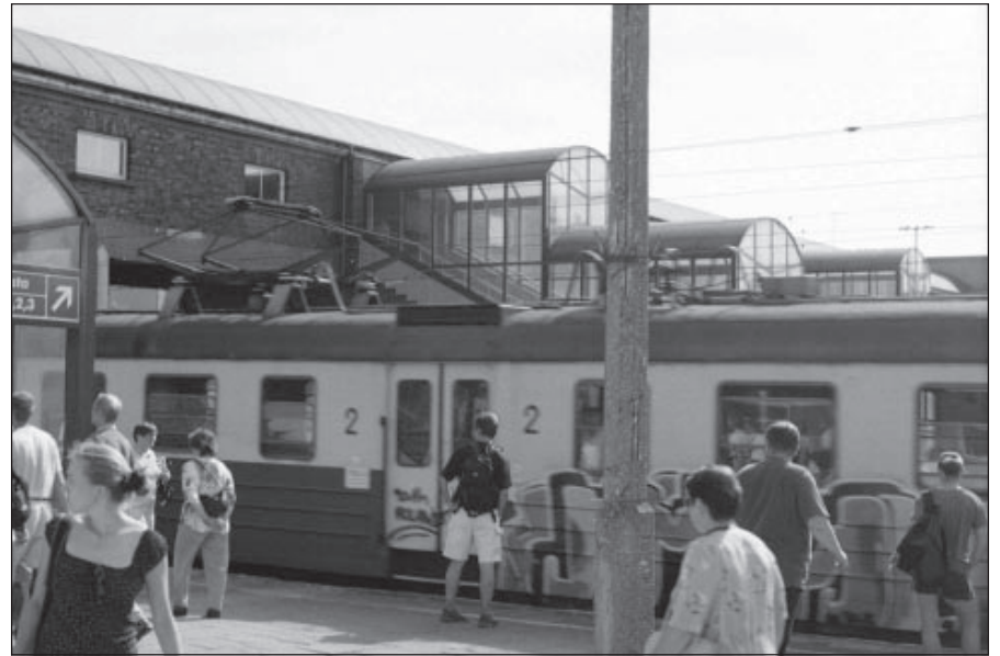
Outlying station with tram loading. Note the overhead walkway to get to the platforms.
